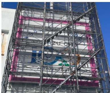
=設置中の様子=
